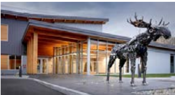
Photo of WLFN's new administration building at Quigly Drive
